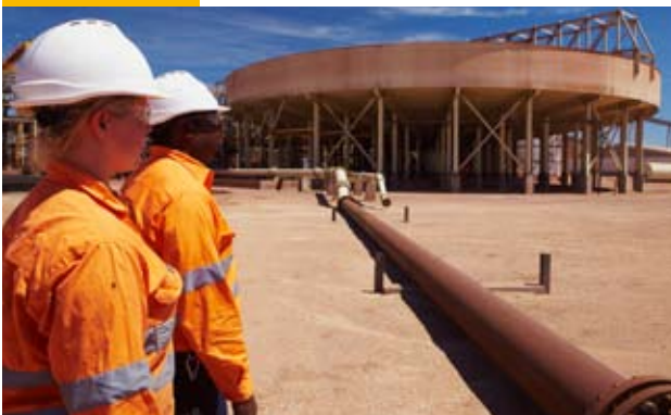
The Prominent Hill processing plant
